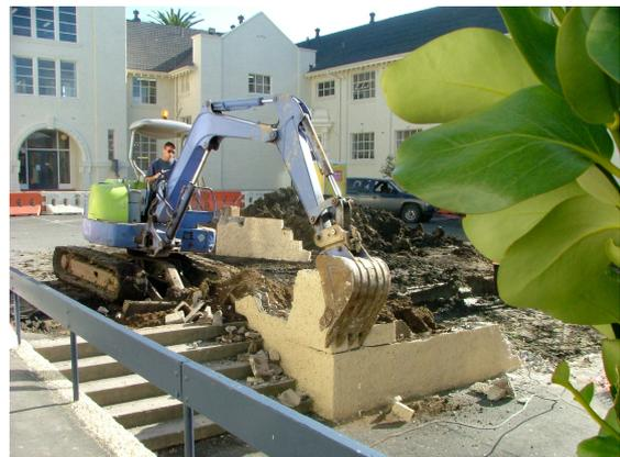
The seating along the tunnel wall was removed and the retaining wall was demolished.
