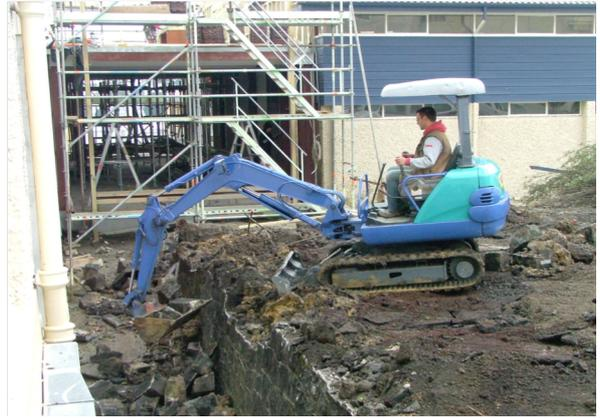
Much debris has been taken away and here new rocks arrive for the new wall. In the other image the wall is well advanced and back filled with rubble.
