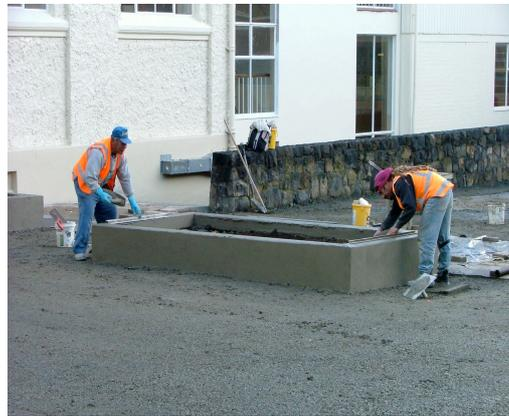
Form-work is in for new paths and the base course is in and rolled, steel work is down and the yellow upturned buckets are the positions of lights which are to be flush with the paths. The image is taken through the earlier large-pane back door to the quad. It had wire safety mesh. In the second image a concrete layer is going in over the base course and is ready to be screeded.
