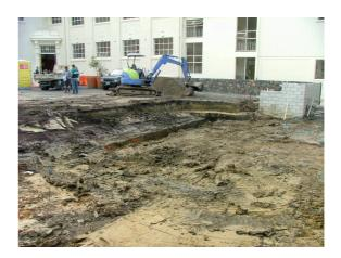
Progress work on the terracing and the first concrete is in. Also in this second, image new blockwork can be seen as can the completed stone wall.
