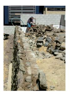
The new wall is higher than the old cut-stone one and here the inside of the new wall is being pointed. One wall is being finished as another, nearby, is demolished.
